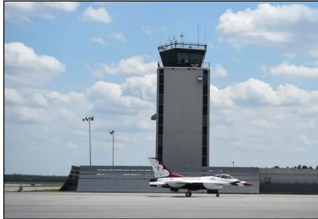
AGS Airport Traffic Control Tower
